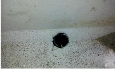
Make the hose sit flush with the inside base. Secure in place with a silicone gun.
